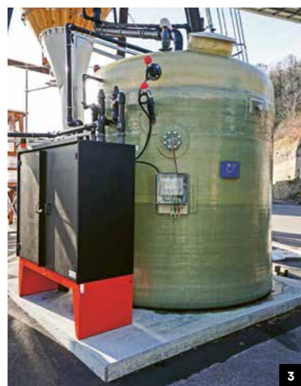
1 Künten (CH), system do rozpuszczania soli Pico 2 Loveresse (CH), system do rozpuszczania soli Basic 3 Fribourg (CH), system do rozpuszczania soli Quanto
